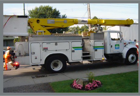
Arrival of BC Hydro crane truck.
